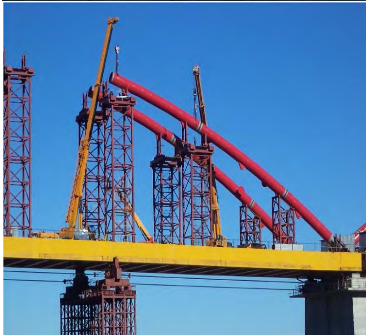
Transportation of the Bridge's Nodes of 110tns
