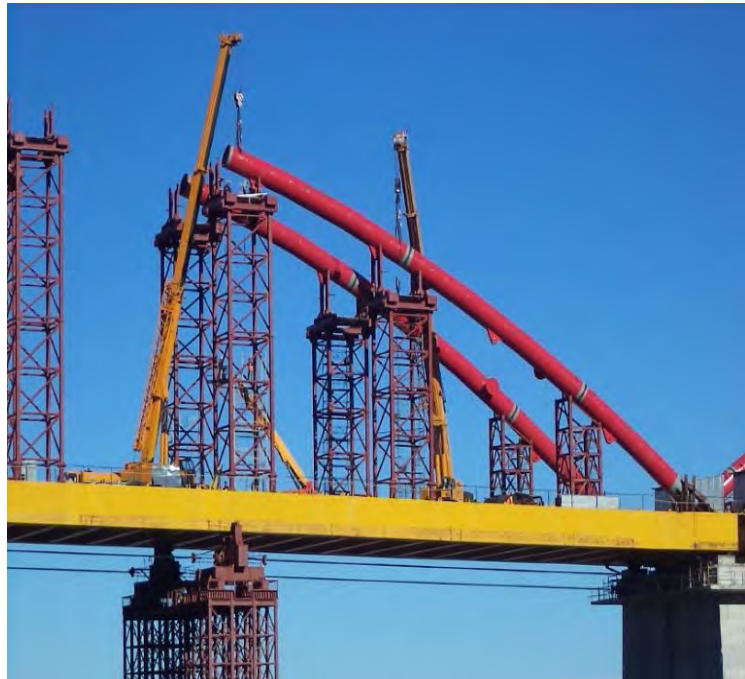
Transportation of the Bridge's Nodes of 110tns
